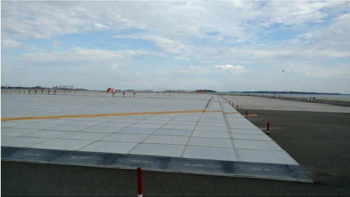
Figure 3 EMAS installation on Boston Logan Departure End of 15R.
