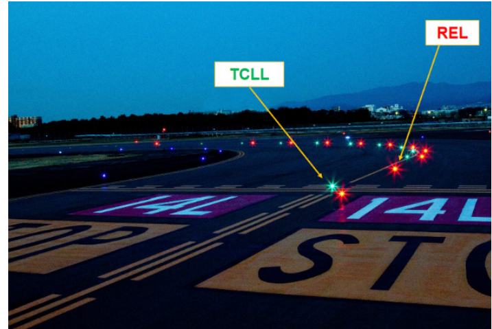
Figure 3 Illuminated Runway Entrance Lights (RELs) (Source: JCAB)
