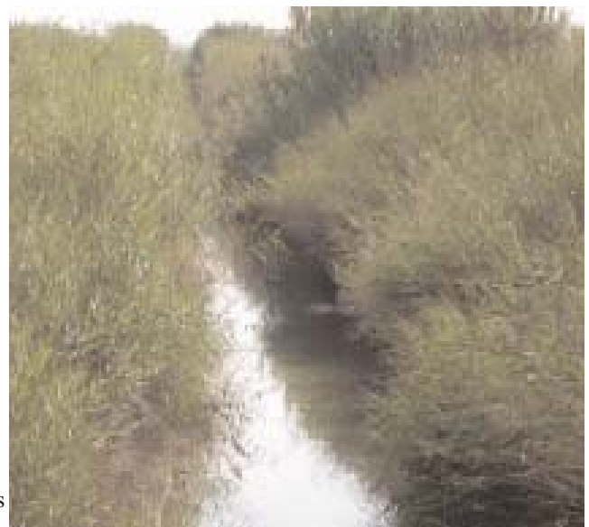
Overgrown ditches like this provide good shelter and nesting cover for hazardous birds
